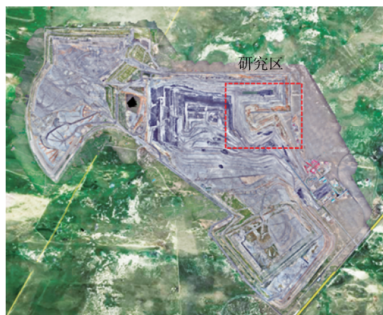
图 1 白音华三号露天矿凸台边坡俯瞰图及研究区 Fig. 1 Vertical view and study area of convex slope of Baiyinhu NO. 3 open-pit mine
